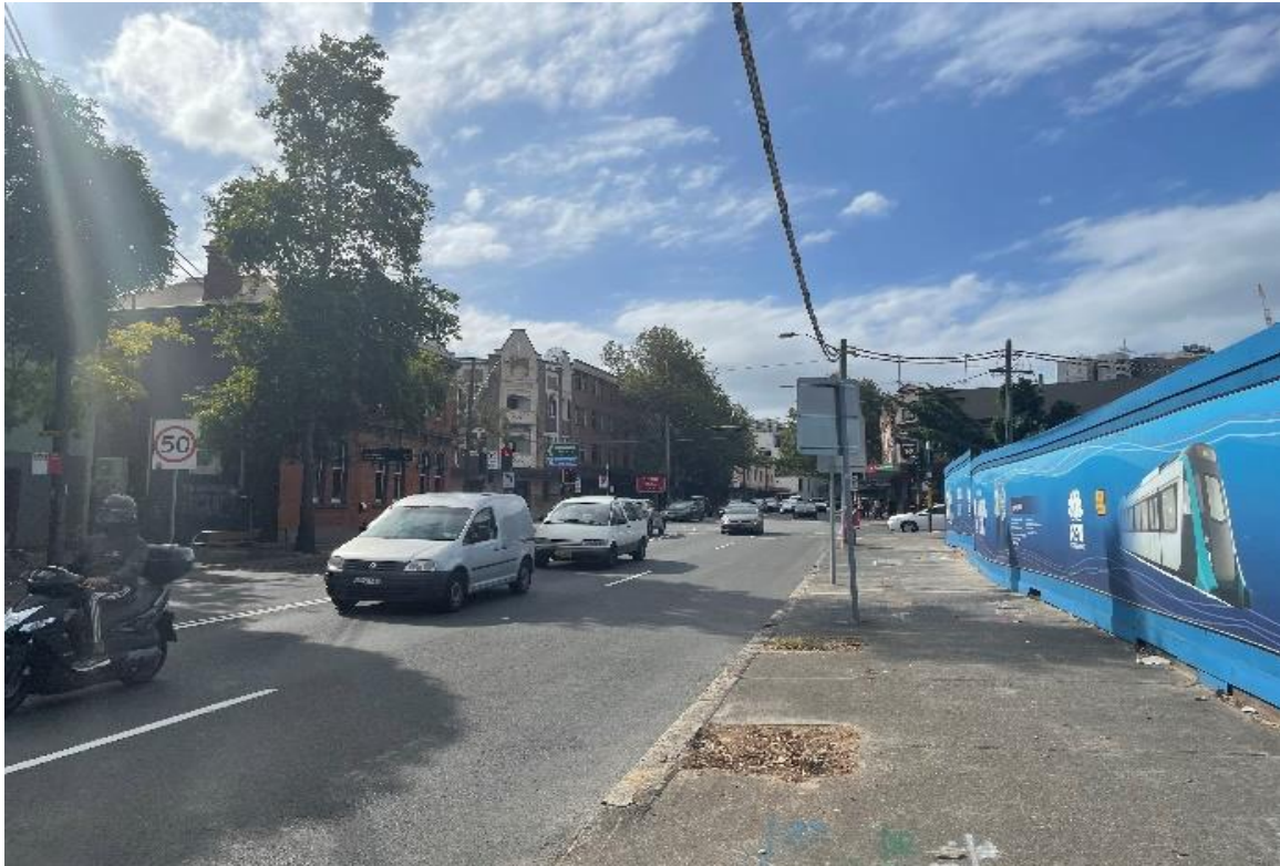
Figure 5: Future Waterloo Metro Station, looking west
